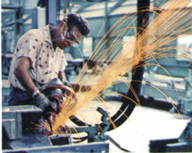
Careful welding of bodies is inspected at many points.
