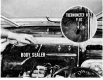
trouble. Just get the thermometers in place again, start the car, and get a new wet-bulb reading. If you find that your delivered air temperature is below the maximum temperature allowable, according to the chart, you've sealed up the leaks that were causing the trouble.
