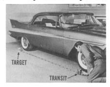
Look down into the transit and move it about until the target is visible. Adjust the range screw until you line up the split image of the target into one unbroken line. Next, turn the dial on the side of the transit until you center the bubble in the level vial. Where the dial stops is your reading in degrees of slope of the floor. This is the figure you will put into the floor-level compensator of each mechanical aimer.
