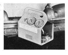
**NOTE:** The 12-volt motorized psychrometer is recommended for air-conditioning service departments. It is faster and more accurate than the inexpensive sling type (Tool C-3668).
