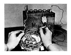
To test for a grounded stator winding, insulate the stator frame from the alternator end frame by placing a block of wood between them. Use a 110-volt test lamp for this test because a 12-volt test may not show up a ground which might occur under heavy load. Touch one prod of the test lamp to
