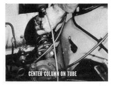
Hold the steering column so it is centered on the tube, and at the same time align the steering column bracket and the column clamp. Carefully examine the coupling disc to be sure there is no distortion or deflection. If there is any visible deflection, move the jacket up or down, as required, to correct the condition.
