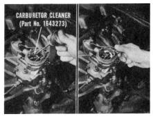
**NOTE:** Do not use oil-base cleaners, or a solvent with graphite or other additives which would leave a film.
