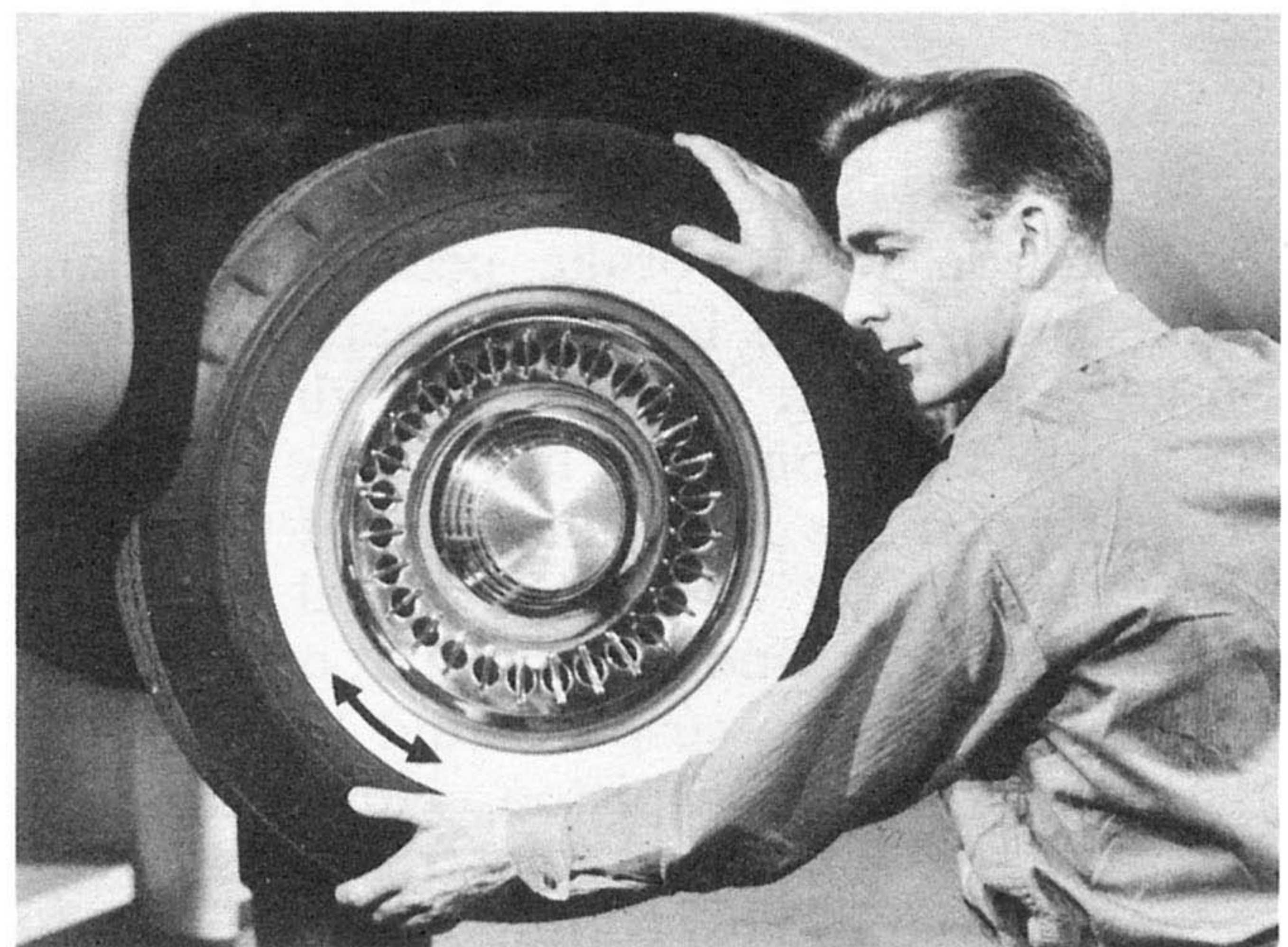
Figure 2—Test for brake drag
