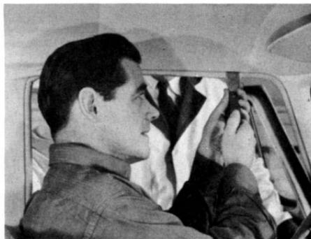
Now you can reinstall the windshield garnish moldings. And, if you find the material at the side a little longer than necessary, trim it so only  $\frac{1}{2}$ " to 1" hangs down below the door windcord. Then, use a dull putty knife to tuck the first and second seam between the roof side rail and headlining retainer.
