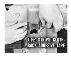
When you install the panel, the switch will fit into the pocket and be protected from moisture.
