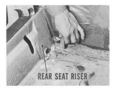
While you're in this neighborhood, it pays to seal inside the rear seat riser on Chrysler and De Soto models. Just reach through the access hole and make a 1" dam of putty inside the outer end of the riser where it joins the quarter panel.
