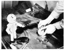
You can connect a new tank unit to the wires and test the panel gauge like you check a single-wire gauge. Just turn the ignition "on" and work the float arm of the new tank unit.
